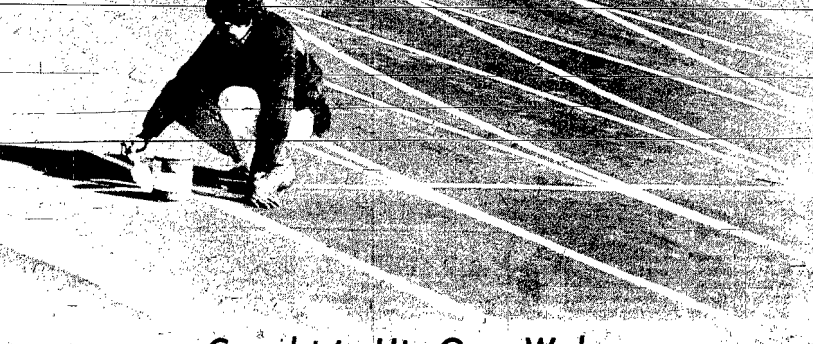
Caught in His Own Web A PAINTER from a Sioux City firm, Keith Julch, seems to be trapped in his own work of painting lanes on the new high school track facilities located near West Elementary School. Both Julch and a fellow worker spent most of Tuesday putting the finishing touches on the eight-lane track, which is expected to see a lot of use when spring practice rolls around.
