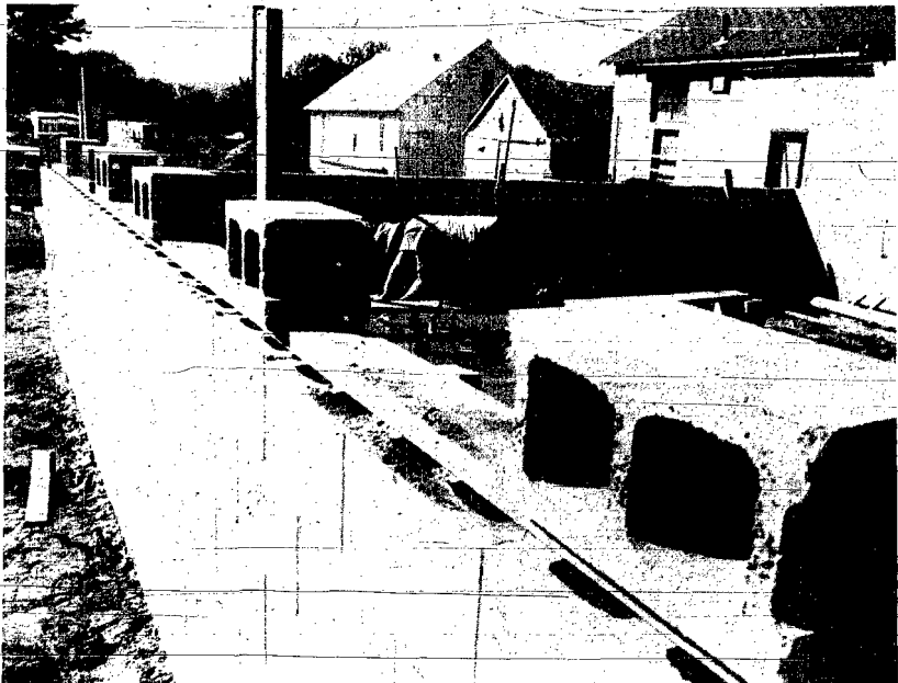
GOING UP PUTTING THE finishing touches on part of a newly-poured concrete floor is Gary Zierke of Pierce who works for Lenz Construction of Pierce. The new floor is part of the construction of a 24 by 36-foot addition to Commercial State Bank in Hoskins. According to bank executive vice president Fred Otten, the new space to the rear of the building will be used for executive offices, director's room and storage vault. Scheduled date to move in the new facility is Jan. 1. In addition to the expansion, the bank is undergoing a facelift in the front. Plans are to expand the present size of the windows, add a night-time depository box and build a single canopy.
